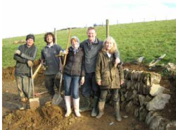
Learners in front of the stone-faced earth bank they've built themselves.
